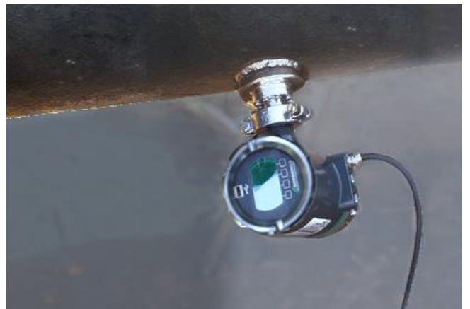
Figure 3: Example of a Weldolet installation
